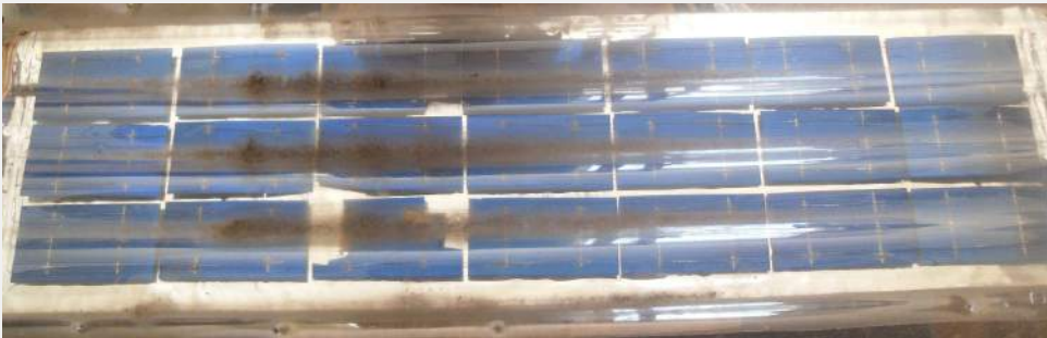
The cells are extremely fragile and are easily damaged by falling braches.
